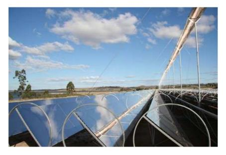
Figure 14: Concentrating Linear Fresnel Reflectors
