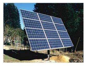
Figure 8: Pole mounted tracking array
